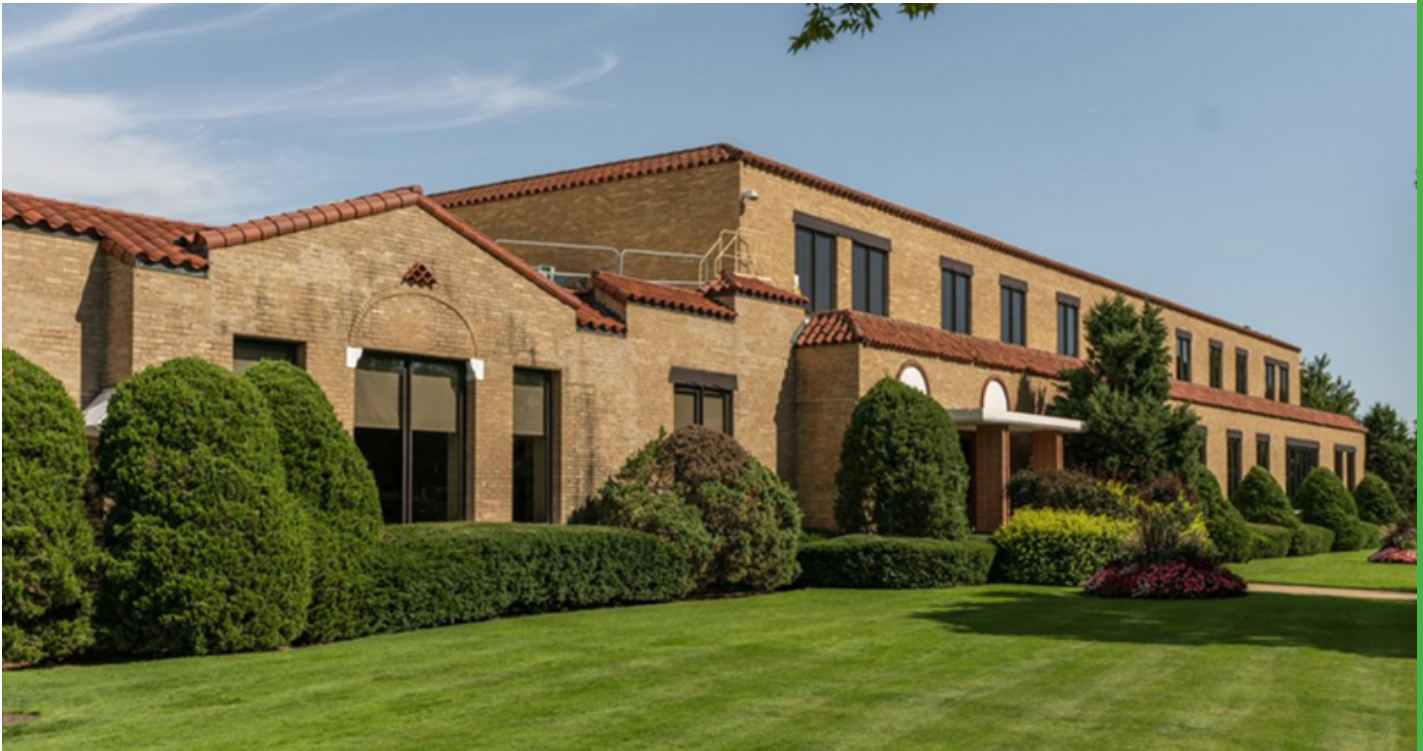
Mars Wrigley Site Building Façade
